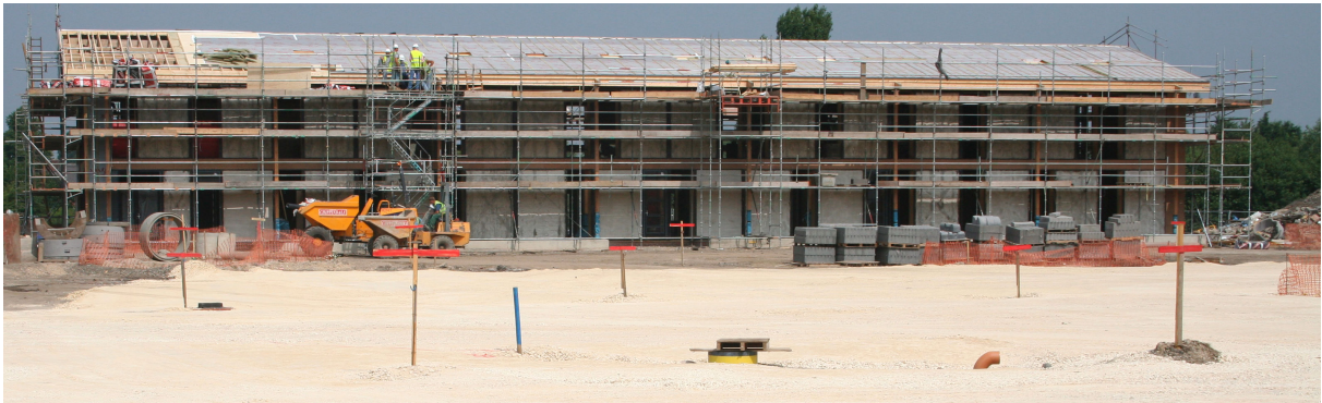
Work on York's Eco-depot October 2006 © Christian Vassie
